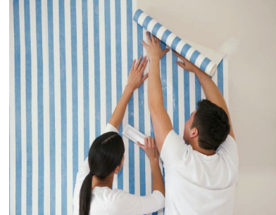
Wall and Floor
